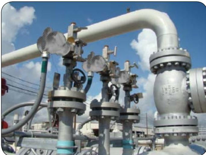
Transmitter isolation valves for pipeline. Pressure Instruments can be used with a transmitter, pressure gauges or pressure switches. Built in manifold eliminates extra valving (5501-00).
